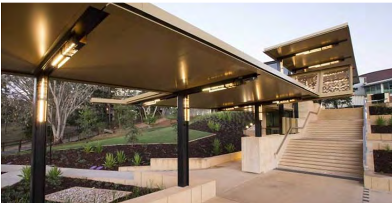
Source: Covered walkway at UQ St Lucia Campus featuring Equideck roofing in COLORBOND steel | Architecture & Design (architectureanddesign.com.au)
